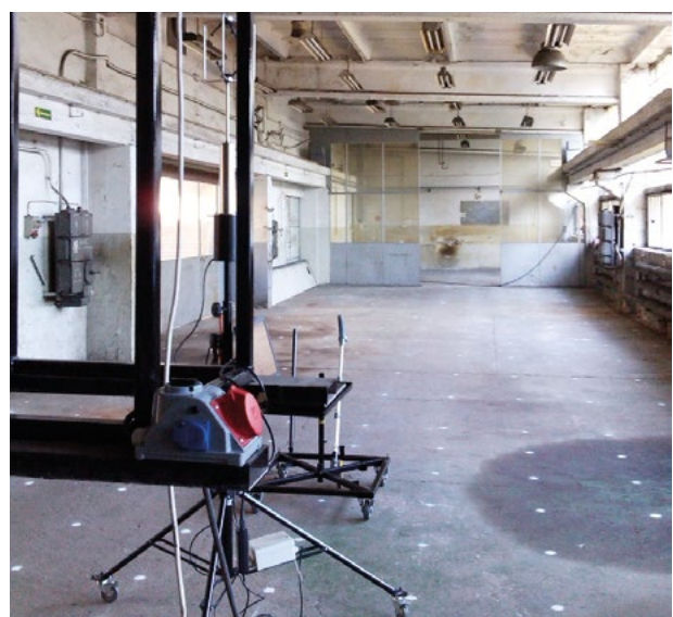
Figure 2. View of the measurement site for testing the jet fan air flow profile
