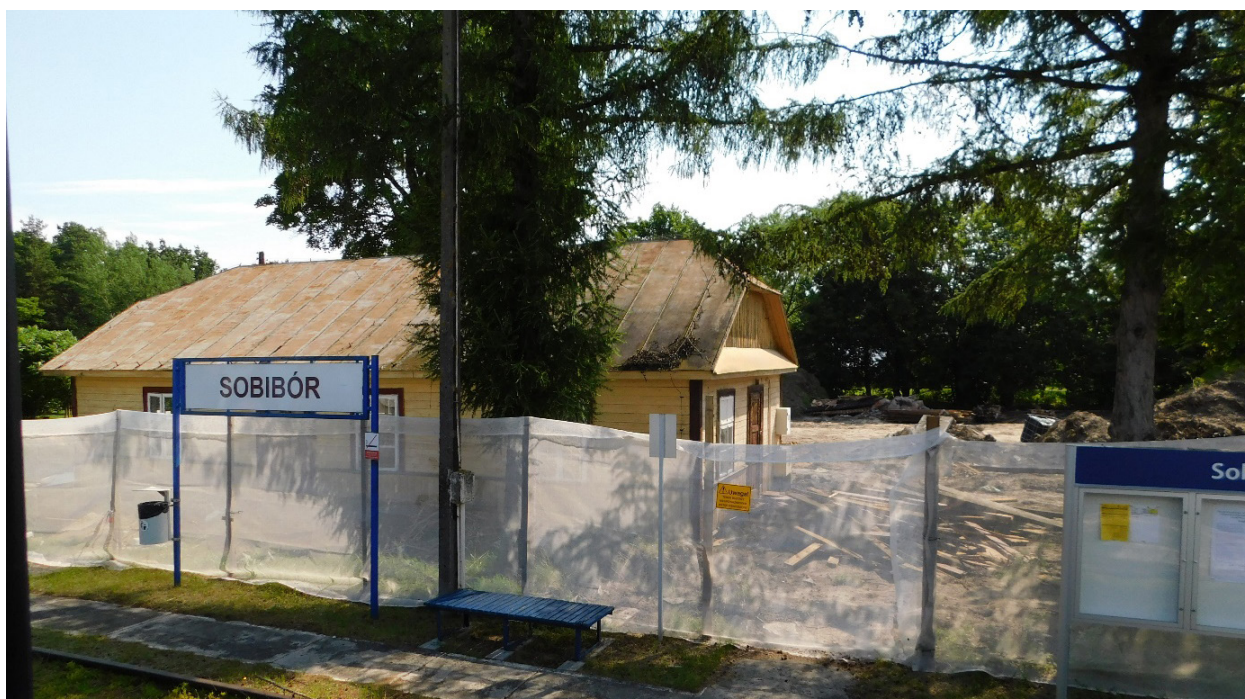
Fig. 9. Renovation works at the Sobibor railway station in 2020.
