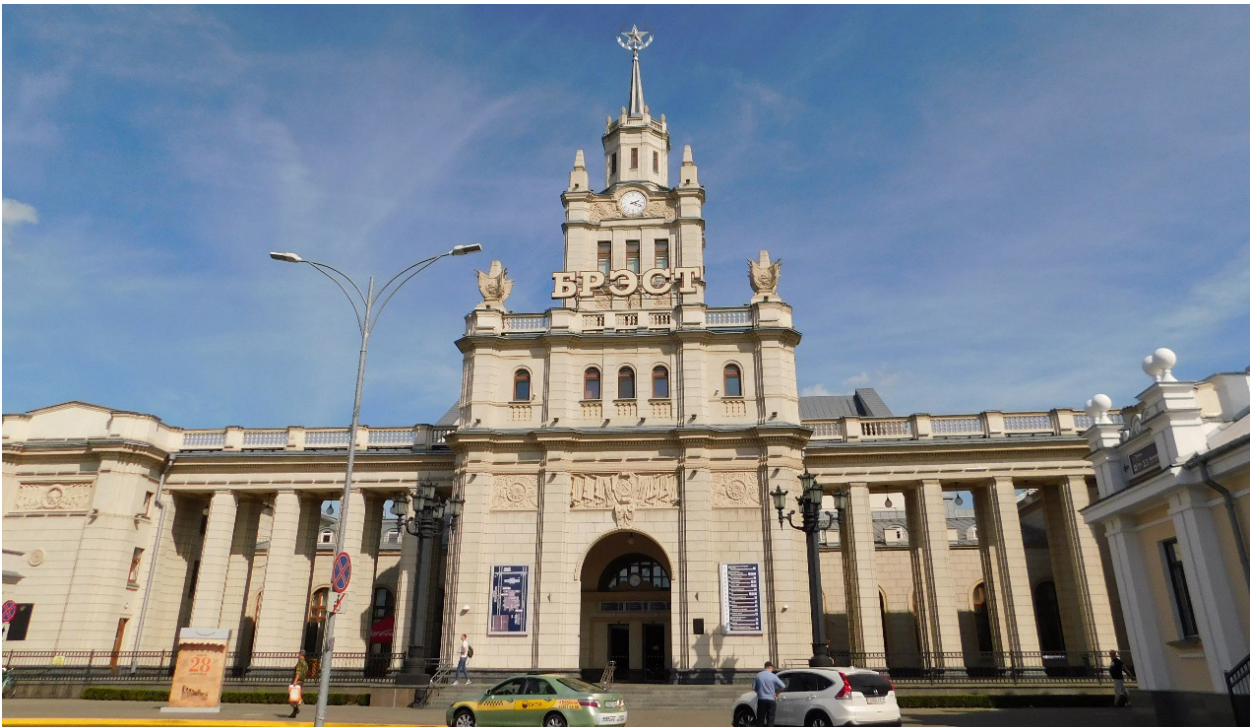
Fig. 4. Railway station Central Brest in 2019.
