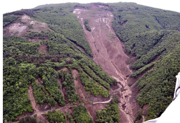
Fig. 2. General view of a landslide formed on the vulnerable slope of the Jokhoniskkevi River, right tributary of the Vere River (photography by Robert Diakonidze)
