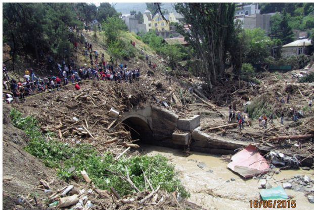
Fig. 3. Oval tunnel positioned under the Vake-Saburtalo motorway and the place of flooding (photography by Robert Diakonidze)
