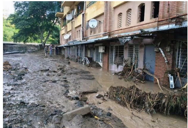
Fig. 5. Flooded settlement territory as a result of broken newly built tunnel (photography by Robert Diakonidze)
