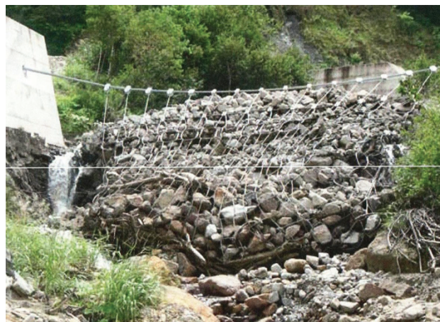
Fig. 6. Construction of lattice type metal networked sediment trap
