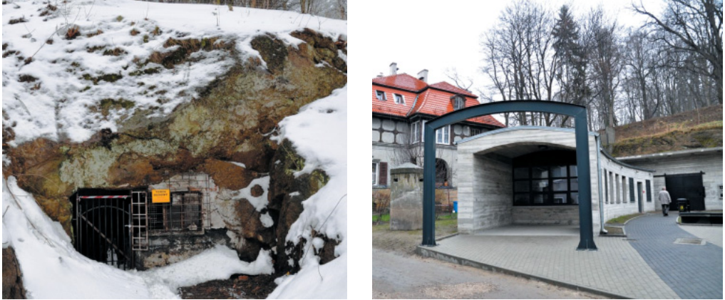
Fig. 9. Tunnel in the Park Mountain in Kamienna Góra- before the restoration work and the entrance to the underground tourist passage
