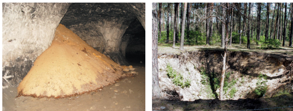
Fig. 6. Caving-in underground the Nagórzycie Grottos and the subsidence on the surface
