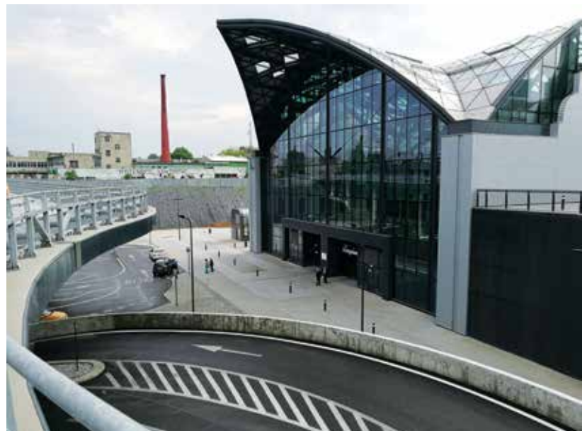
The new station Łódź Fabryczna: east entrance
