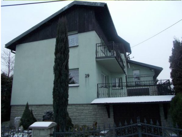
Fig. 1. The walls of the building as an extension of the foundation walls (Foto: M. Buško)
