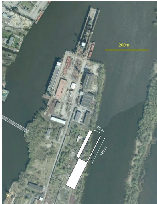
Figure 1. Analyzed area with approximate positions of loading quay, gantry and dolphins indicated. Source: Authors based on Google Earth.
