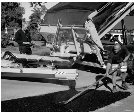
Fig. 11. Work using SPRIDER (from the authors' collection).
