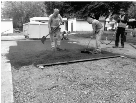
Fig. 4. Partial repair using a conventional hot box (from the authors' collection).
