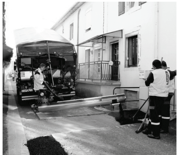
Fig. 8. SPRIDER range [7] and operation in tight spaces (from the authors’ collection).
