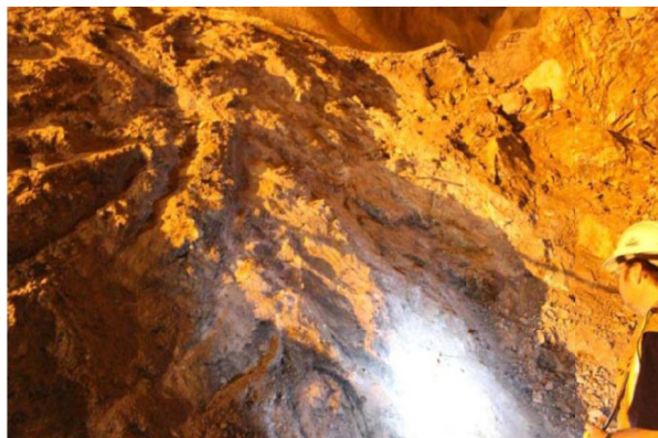
Fig. 3. Shear zone exposed after failure
