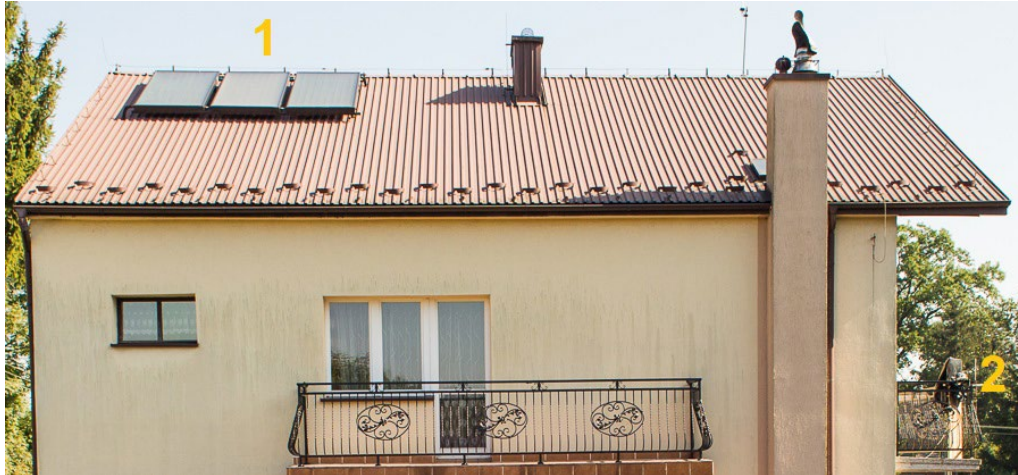
Fig. 2. Analyzed building with solar collectors (1) and solar radiation density meter (2). This picture shows the south-west side of the building
