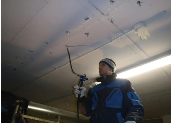
Fig. 10. Crack sealing at site 8
