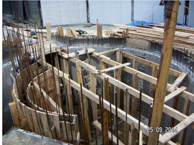
Fig. 5. Przemyśl – implementation of the underground rotunda - the entrance to the underground tourist route (photo by UM Przemyśl)
