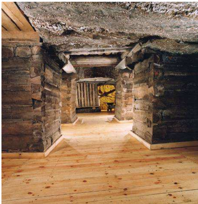
Fig. 6. XVII-c. chamber "Mysiur" in KS Bochnia secured In accordance with conservation requirements (photo by J. Chmura)
