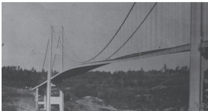
Fig. 1. Flutter of Tacoma Narrow Bridge
