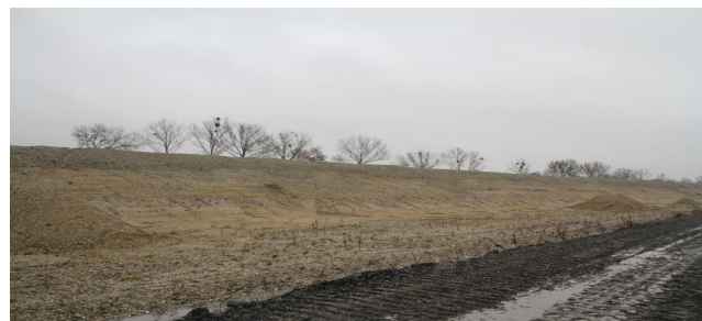
Figure 3: Fragment of the dam built of material from local mines, km 1+900.
