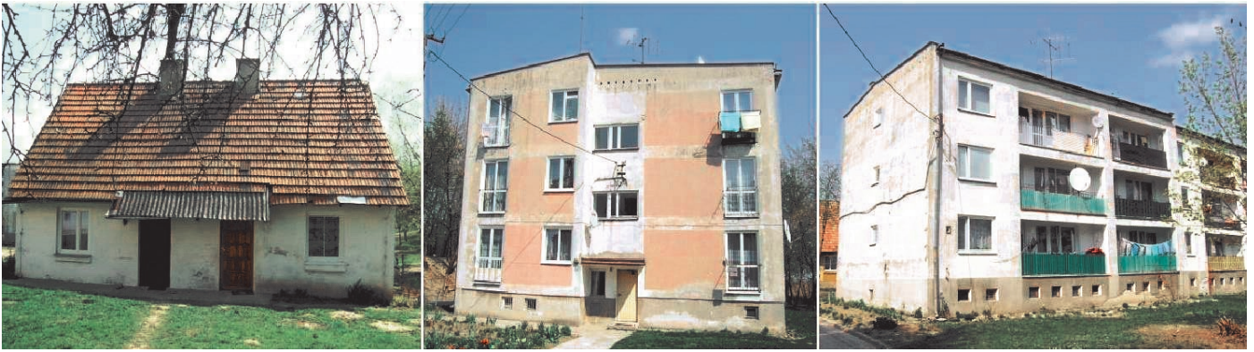
Fig.2 Buildings before the investment: two-family, one-staircase and two-staircase dwelling-house [15]
