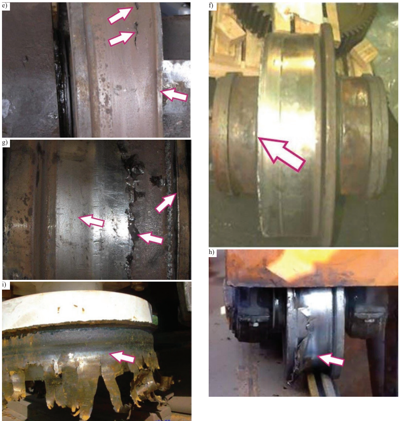
Fig. 2. (e–i) Examples of typical damage of crane vertical wheels and horizontal guiding rollers
