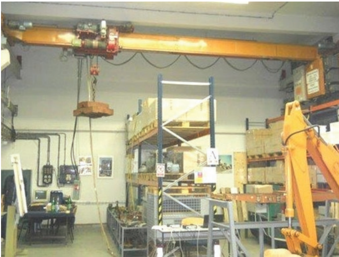
Fig. 4. Measurement of lateral forces acting on the wheels of a single-girder bridge crane
