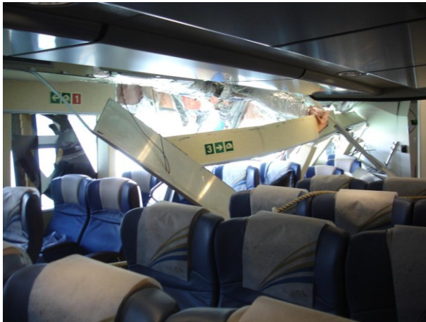
Fig. 2. The damage of passenger compartment on the starboard side of the HSC The Cotai Strip Expo [9]
