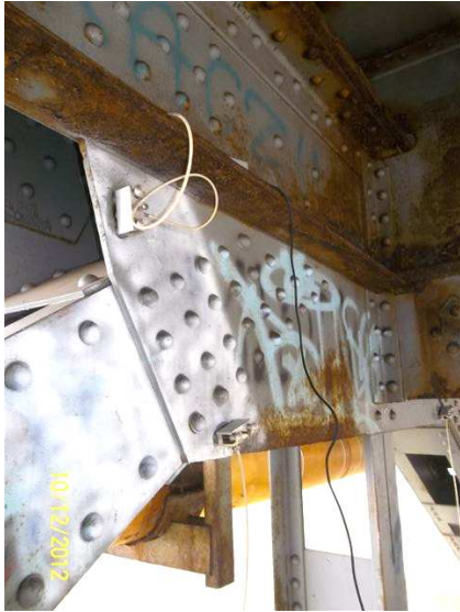
Fig. 7. Acoustic sensors mounted on the gusset plate of the critical diagonal
