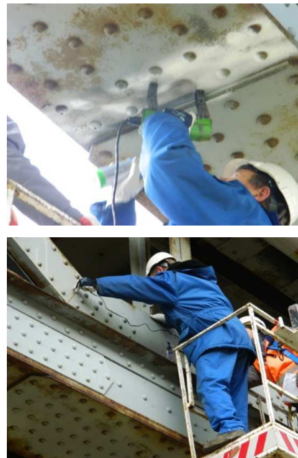
Fig. 8. The qualitative NDT inspection of the critical members and cross-sections
