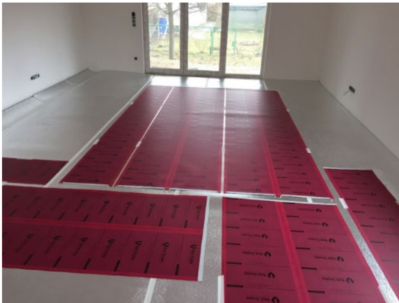
Fig. 1. Red Snake heating film underfloor installation Source: own photo
