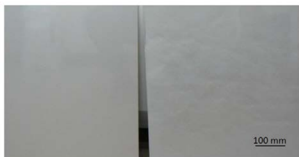
Fig. 3. Cloud defect on coating.
