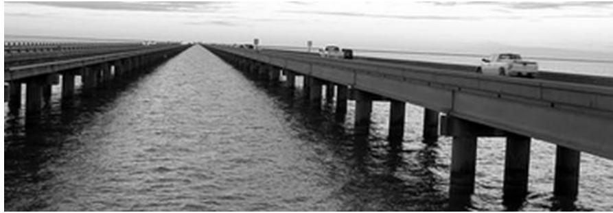
Fig. 1: View of the prefabricated Lake Pontchartrain Causeway bridge in the United States ( http://mapio.net/s/13360936/ )
