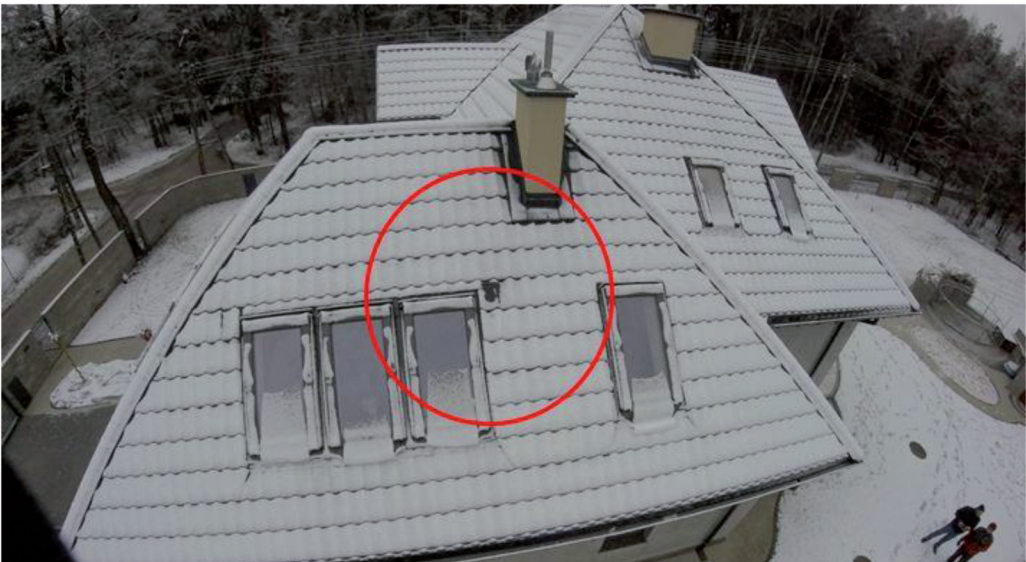
Figure 10. Roof windows, shot from the north. Visible little thermal bridge close to the third window, in the right upper corner – lack of snow [zdj. T. Sasin, 2014]
