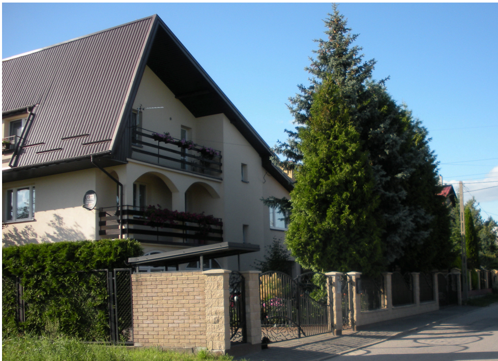
Photo 1: Detached house with different angles of slope – little bit reminiscent of saltbox form of a roof (photo: E. Koźniewski)
