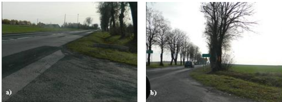
Fig. 5. Limited visibility caused by: a) an unfavorable vertical profile of the main road, b) location of road signs and roadside trees
