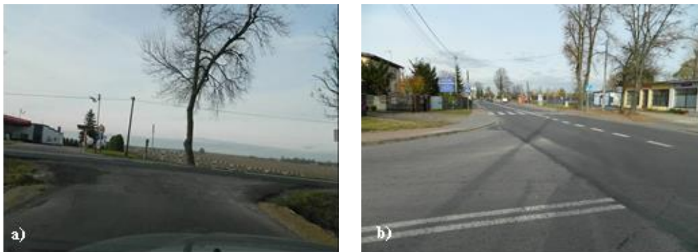
Fig. 6. Intersections: a) with uneven surfaces, b) with a correct horizontal visibility field
