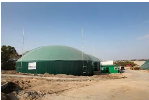
Fig. 2. Biogas plant in Siedliszczki Source: [22]
