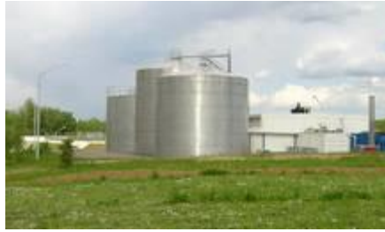
Fig. 3. Biogas plant at the dairy in Ehrmann in Russia Source: [24]
