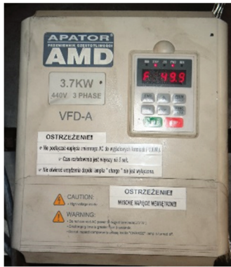
Fig. 7. The equipment used during testing: the electric inverter (coolant pump speed control)
