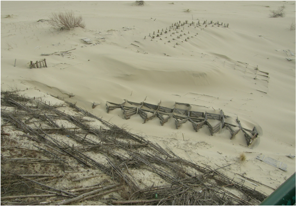
Fig. 12. Stabilisation of quicksand on the Curonian Spit
