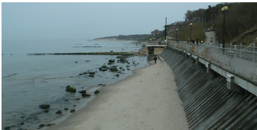
Fig. 9. A massive permeable revetment with pavement on top in Pionerskiy, built in 2008 (570 m long) and extended by 1 km eastwards in 2011
