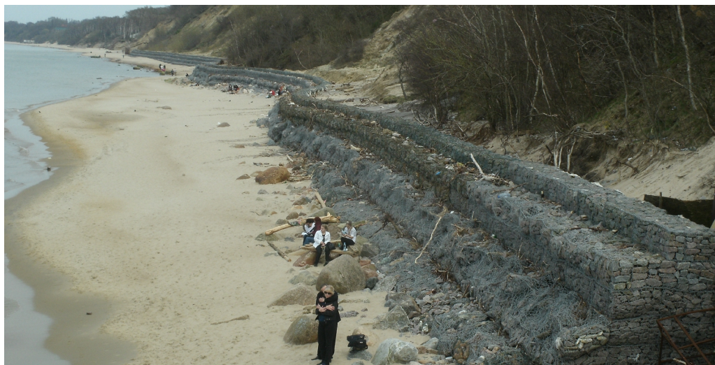
Fig. 8. Gabion structures near Svetlogorsk built in 2009
