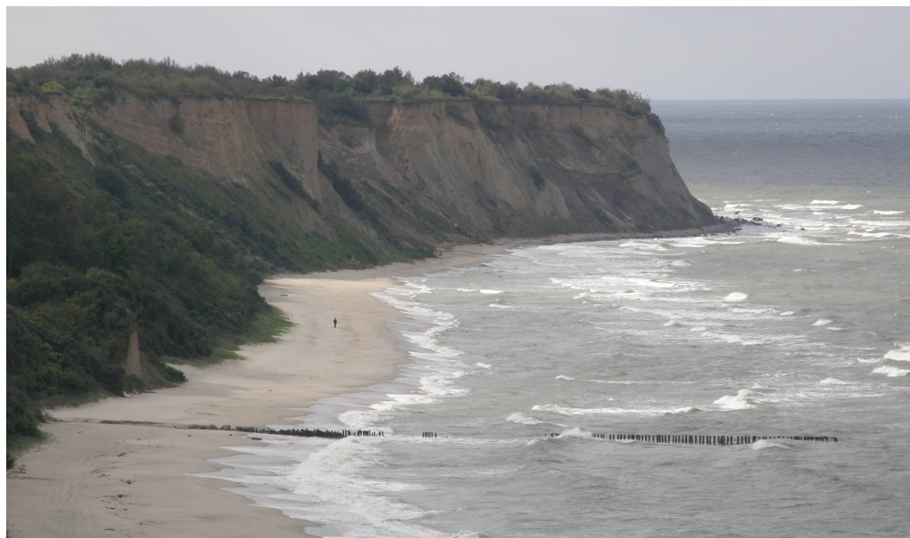
Fig. 6. The single groin near Donskoye (northern part of the western coast of the Sambia Peninsula) constructed in 1938 for protection of the wastewater pipeline outlet
