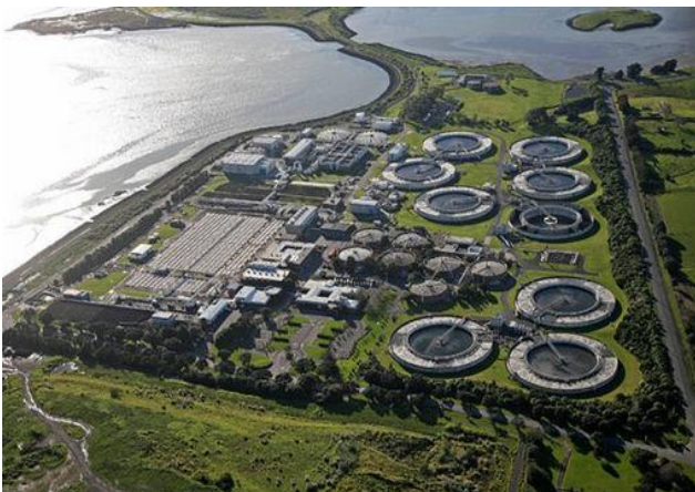
Fig. 1. Shore based Reception facilities look like land based water treatment plants with holding tanks for treatment of received untreated ballast water from ships. Source [3]
