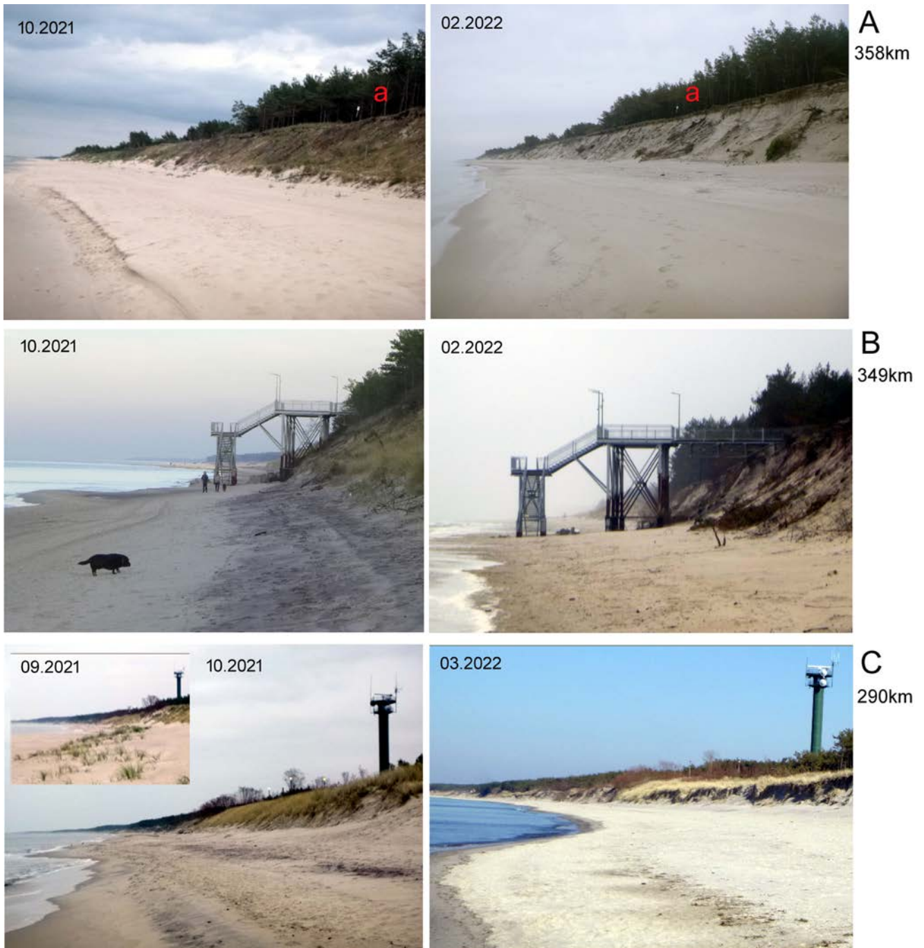
Fig. 13. Comparison of coast retreat after smaller surges in Autumn 2021 and big Nadine in January 2022 on the West coast. Photos from 10.2021 show the coast after Hendrik & Rudolf surges in October 2021. A – lowered beach and then retreat of 3–5 m of a dune toe on the Rega River Sandbar, km 358, a – kilometrage sign. B – lowered beach with heavy minerals and then dune retreat of 6–8 m on the promontory on the Resko Lake Sandbar, km 349. C – embryo dune erosion after October surges, then dune retreat 2–3 m after Nadine surge, Jamno Lake Sandbar, km 290.
