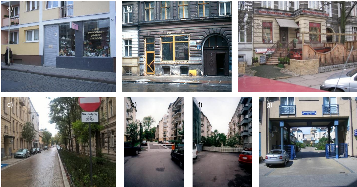
Fig. 4. Impact of mobility on relations between the street and ground levels of buildings. Examples of making ground level “public” in residential buildings (a,b,c). The change of functions at the ground level to control a public street and at the same time benefit from accessibility and proximity of sidewalk. Examples of street functions being “privatized” by: (d) rebuilding and narrowing the street and introducing an (asymmetric) green strip that isolated from apartments, (e,f) closing a section of a street to public access, (g) limiting free access to gated housing estate. Source: Photographs by the author
