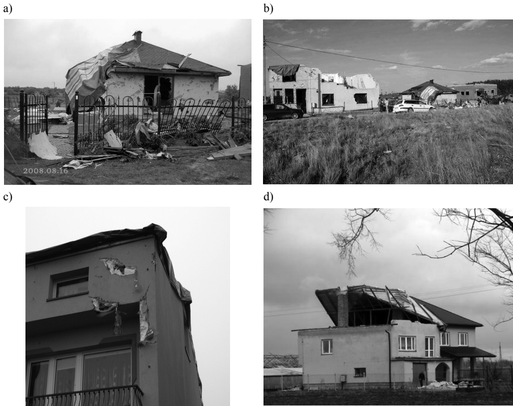
Fig. 17. Typical examples of damage to houses caused by tornadoes in Poland; a) damage to the building of frame construction, b) partial removal of the 2nd storey of a building (Phot. G. Beblot), c) damage to walls inflicted by windborne debris, d) failure of a sheet metal roof.
