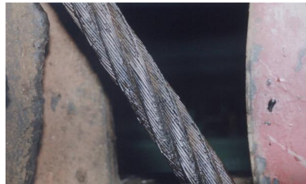
Fig. 7 View of a rope section with fractured wires between the cable wheels of the P4-GIG-2 fatigue testing machine
