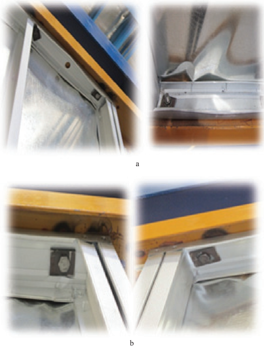
Figure 9. Failure modes of specimens type II a. Top and bottom local buckling; b. tearing of the bottom track's flange b
