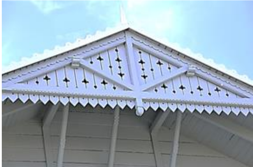
Figure 7. The gable decoration is made of boards with a decorative motif
