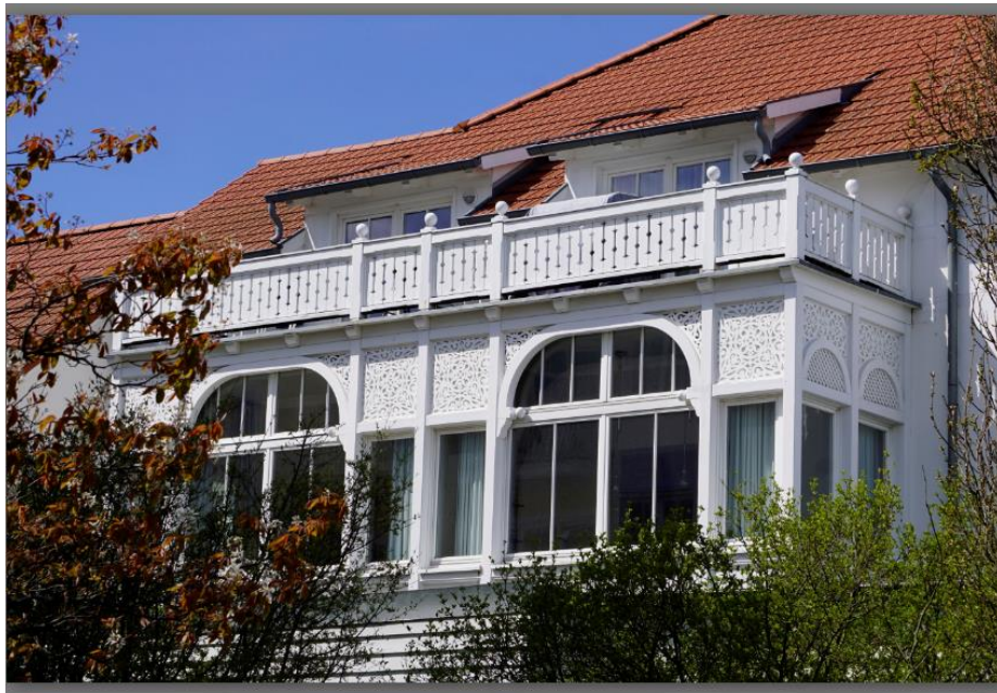
Figure 4. Porches and balconies of wooden structure filled with openwork panels Murkanerstrasse 1
