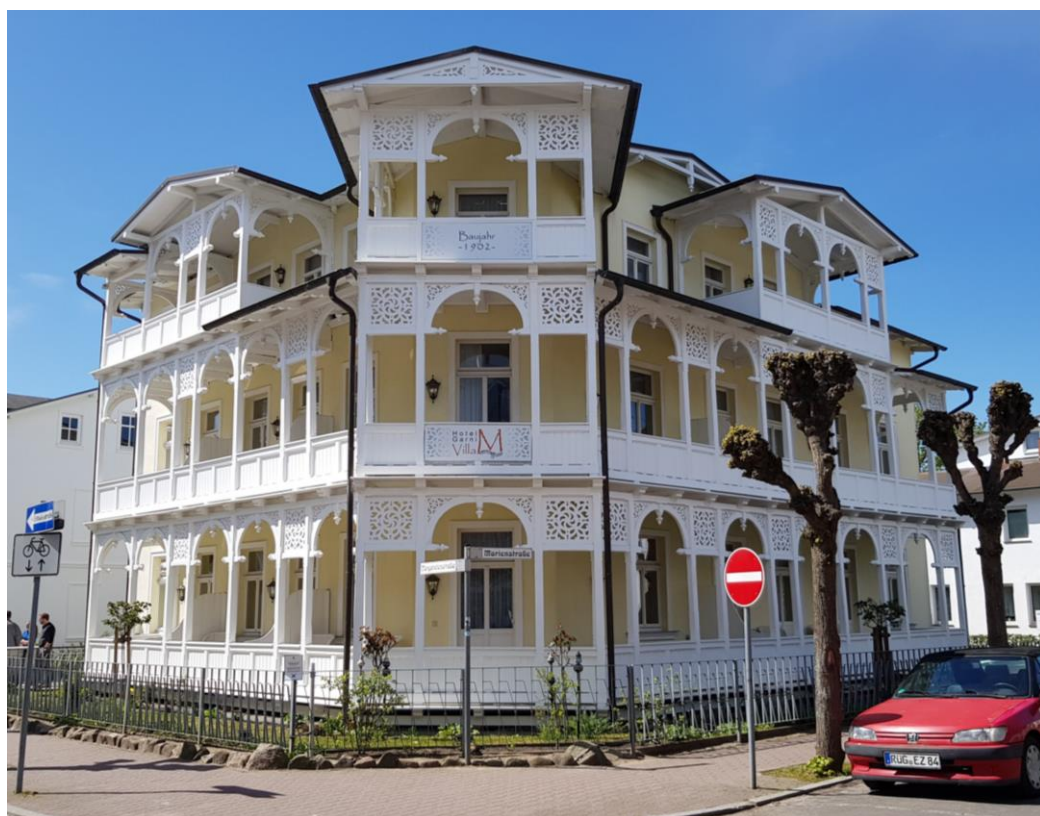
Figure 6. Construction of balconies and decorative panels in Villa Meeresgruss on Marienstrasse 1
