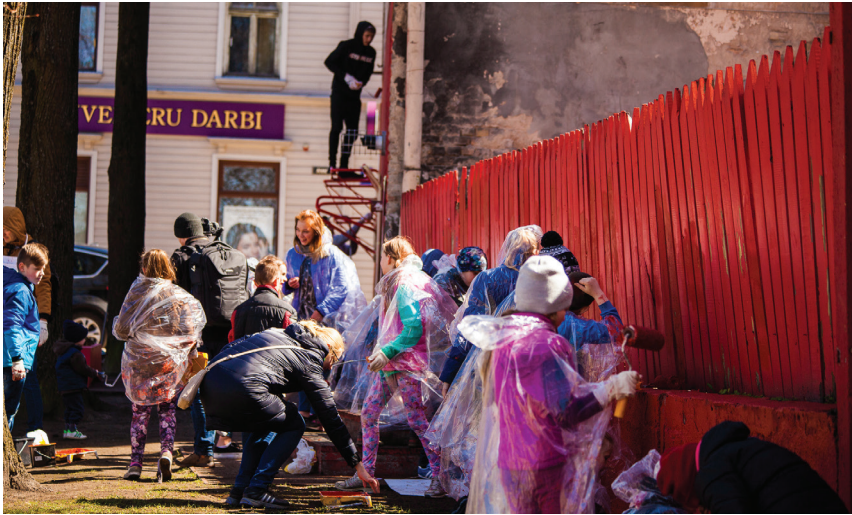
Image 6. Laba Vieta (eng. Good Place) movement – public-driven urban upgrade. Work in progress. Alekša Skvērs, Sarkandaugava, Riga [19]
