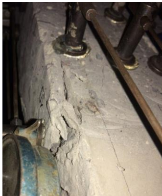
Fig. 5. General view of a fracture of damaged samples BD-3 and BD-4
