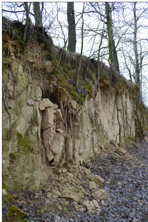
Figure 2. Loess falling off vertical slopes of the gully
