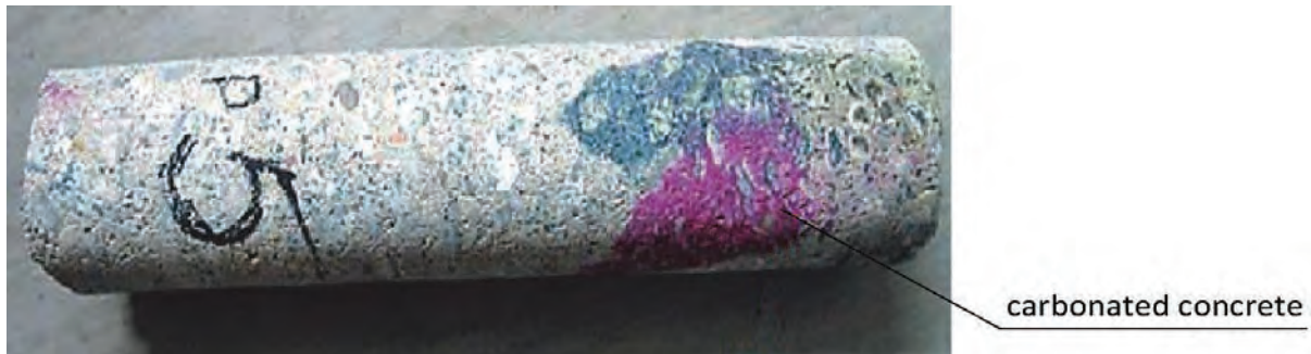
Fig. 18. A view of the core bore with marked carbonated concrete that was evaluated using the rainbow test, according to [37]
