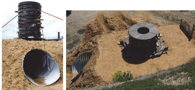
Figure 1. View of tested culvert
