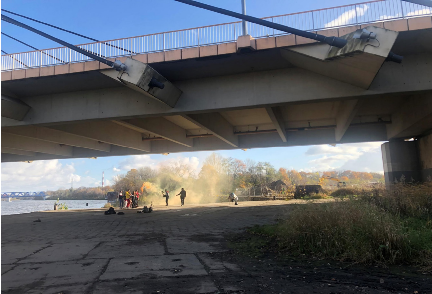
Fig 7. Movie makers working on a video clip in the surroundings of the flyover construction elements in the area of the study. Milenijny Bridge (left-bank flyover) – span № 8, between 8 th axis and Odra river bank, 20.11.2020. Source: author's Elżbieta Komarzyńska-Świeściak own photo archive
