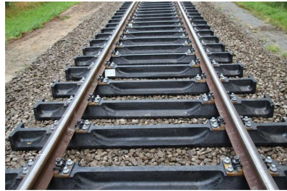
Fig. 1. Polyethylene railway sleepers
