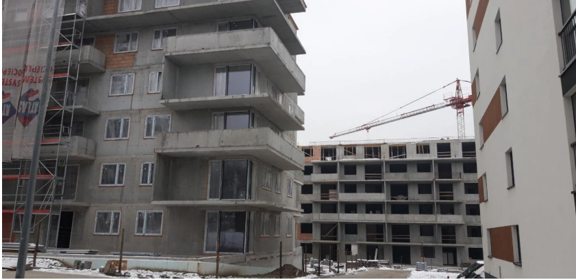
Phot.1. View of the project site
