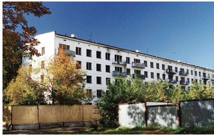
Fig. 1. Moscow, 2002. Building at 8 Khimkinskiy Bul'var before modernization [15]
