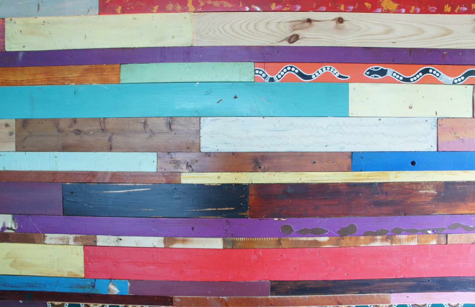
Fig. 2. Wooden panels reclaimed from demolished buildings and incorporated as wallcovering in a new location. Restaurant and music club situated in the complex La Cité de la Mode et du Design, Paris, proj. D. Jakob, B. MacFarlane; photo by the author, 2017
