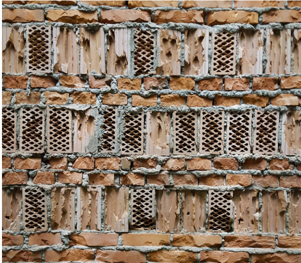
Fig. 3. Bricks reclaimed from demolished walls of refurbished building and used as finishing coating of inner multilayered wall separating main auditorium from lobby. Centrum Spotkania Kultur, Lublin, proj. Stelmach i Partnerzy Biuro Architektoniczne; photo. by L. Nyka, 2017
