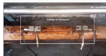
Fig. 2. (a) Example of 11-day itinerary of the ship, (b) Distribution of sensors onboard ship, (c) Monitoring system on the bridge, (d) Flowmeter clamp-on sensors in the machinery room
