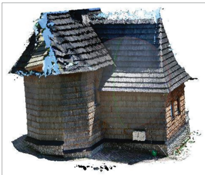
Fig. 9. Model of the south-western wall obtained using the UAV
