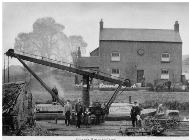
Fig. 6. Crane for handling between the mean of rail and water transport, the unloaded carts in the background [8]
