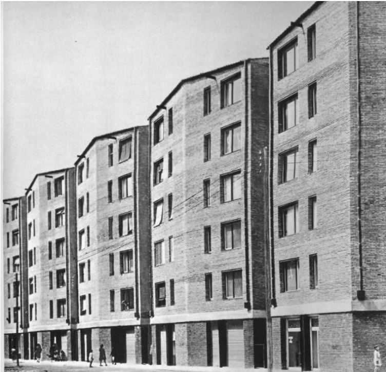
Fig 12. MBM social housing in Calle Pallars, Barcelona. Source: [24]
