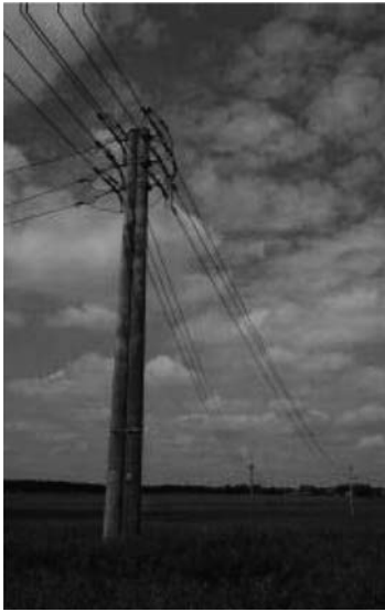
Fig. 1. Spin-cast pre-tensioned concrete electric power pole [3].
