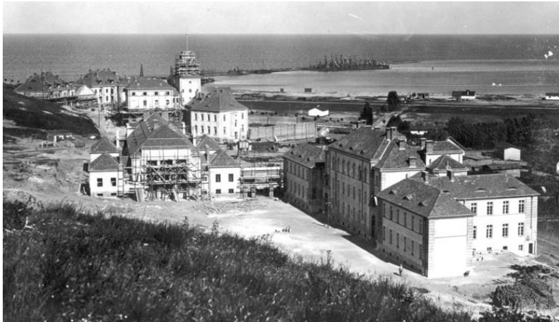
Fig. 13. Gdynia Oksywie — view, from above, of the barracks under construction and provisional harbor with wooden piers: south and north, 1926 [Navy Museum Archives]
