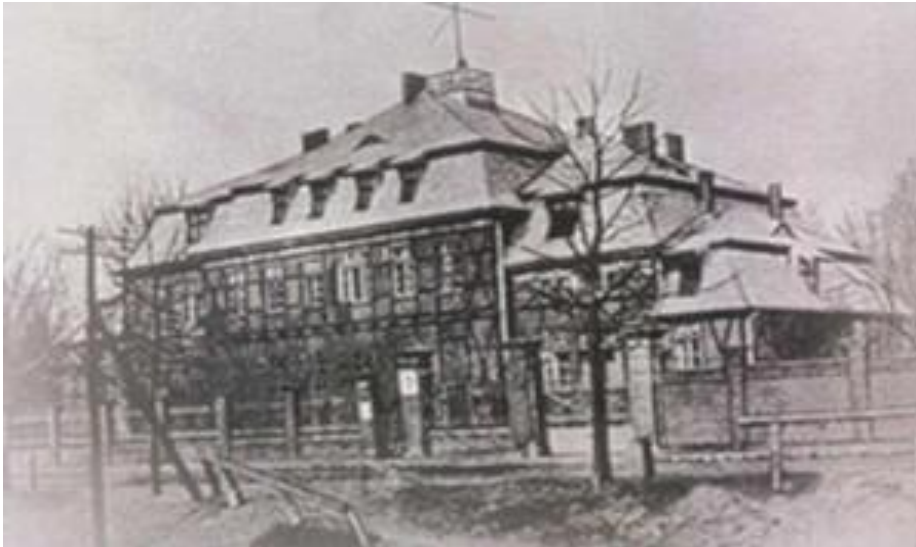
Fig. 1. The building of the former officers mess where the Provisional Instructor Courses for naval officers were run [8, p. 62]
